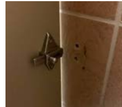
Non-functional cubicle doors and locks
