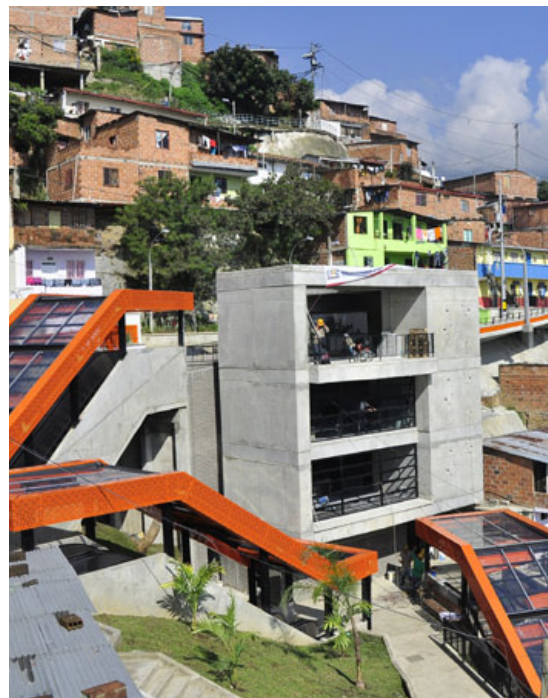
PART OF THE NEW METROPLÚS SYSTEM IN COLOMBIA.
